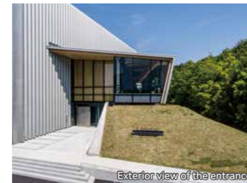
Exterior view of the entrance A ramp is provided at the entrance to ensure barrier-free access
