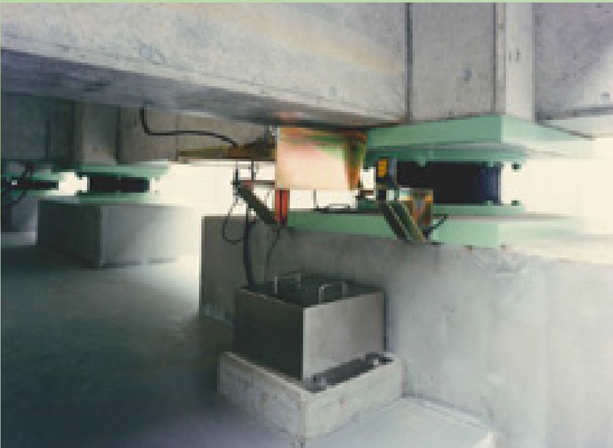
▲ Seismic isolation layers and devices
