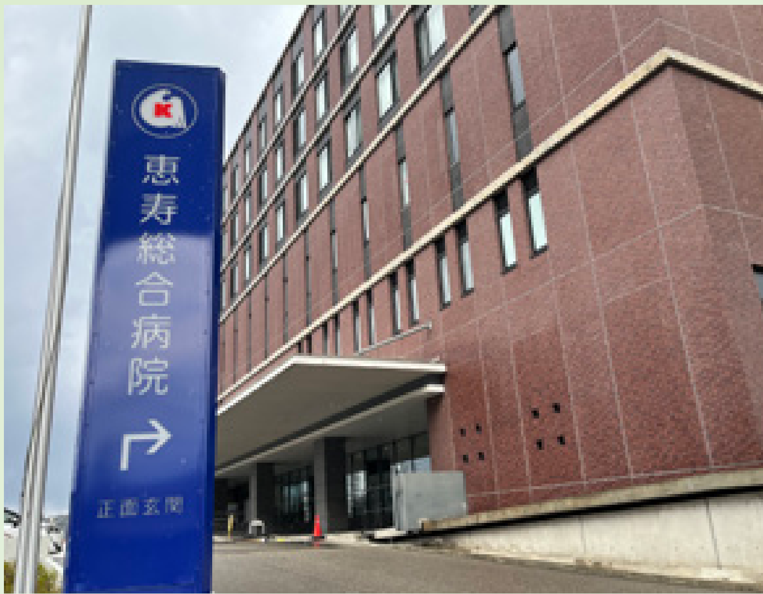
▲ Appearance after the quake
