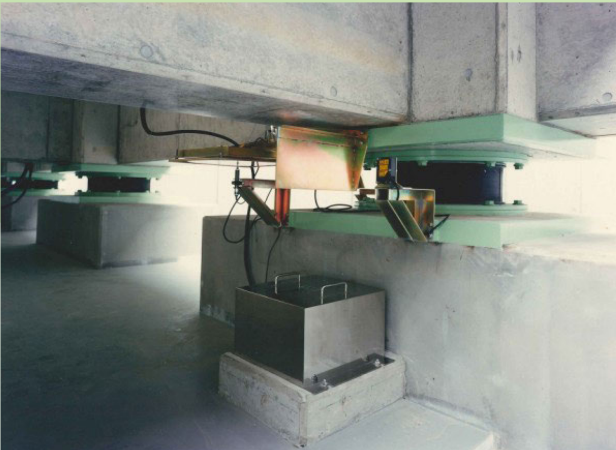
▲ Seismic isolation layers and devices
